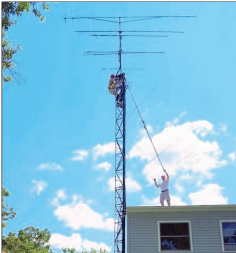
That is W3GAD on the roof, positioning the 6 meter beam for KA3WXV prior to the final raising to the mounting position on the mast.
